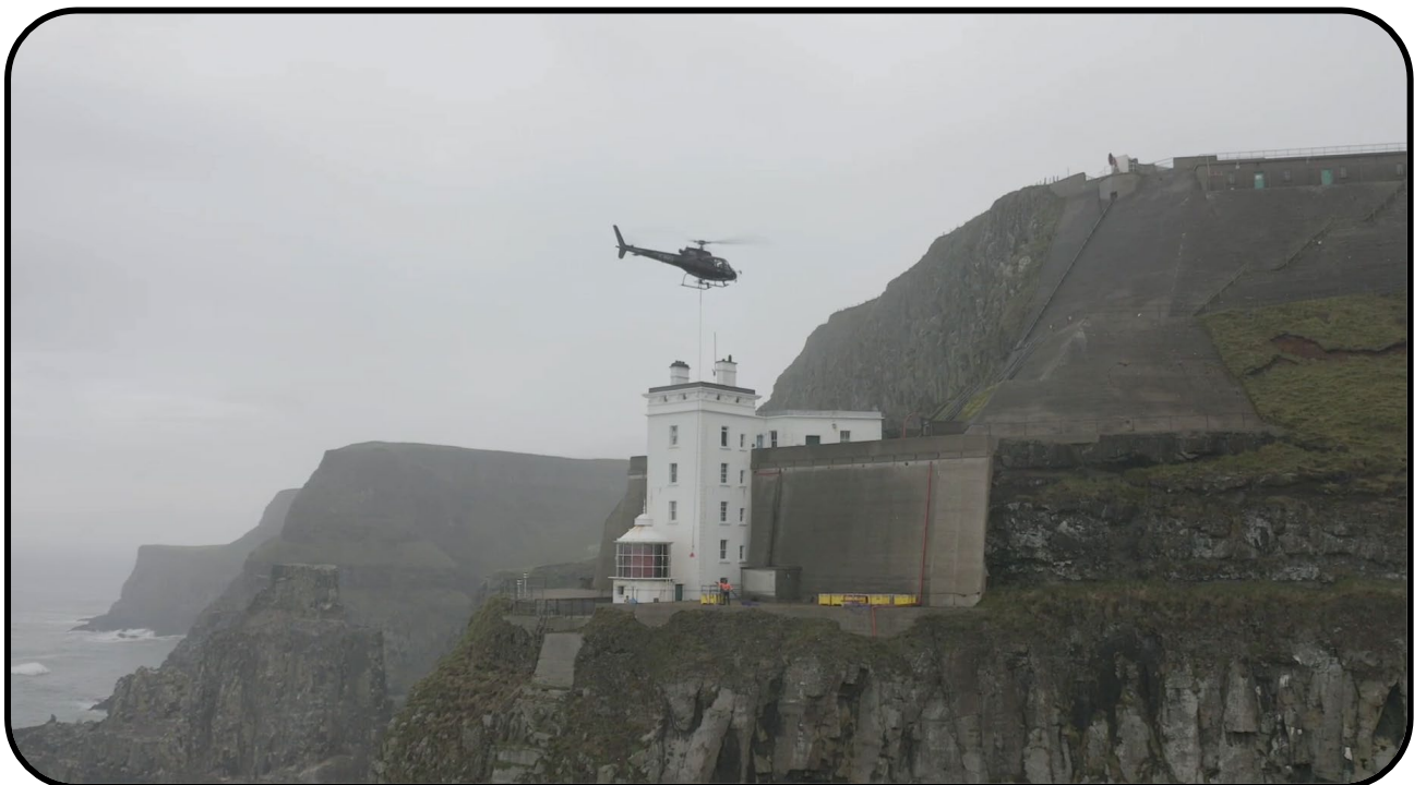
Figure 11: Delivery of new materials and removal of old from Rathlin West with heavy lift helicopter
