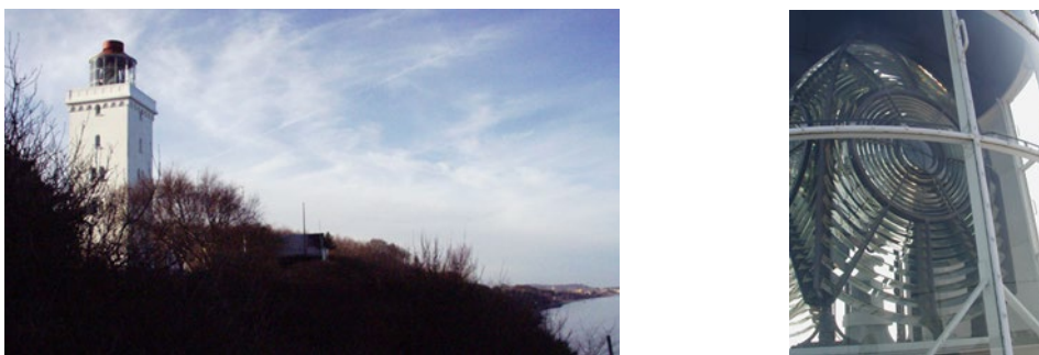
Figure 5: Nakkehoved Lighthouse, at left the building structure and at right the first-order catadioptric Fresnel lens.
