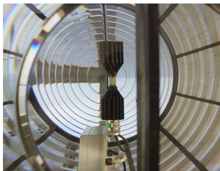
Figure 1: LED light installed in traditional optics
