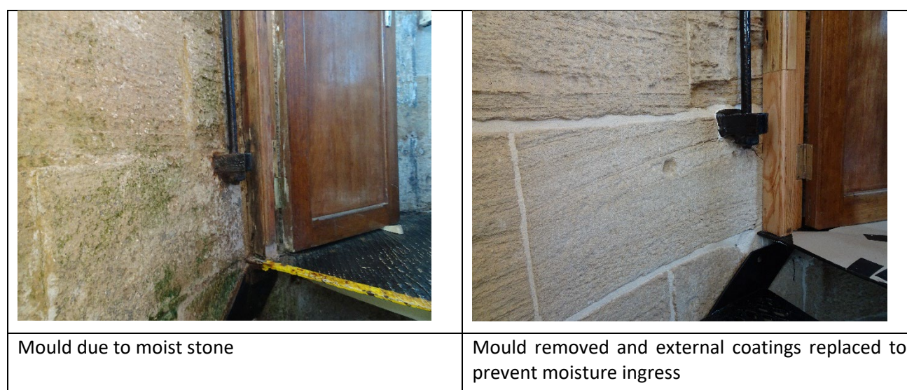
Figure 3: Stone issues and rectifications
