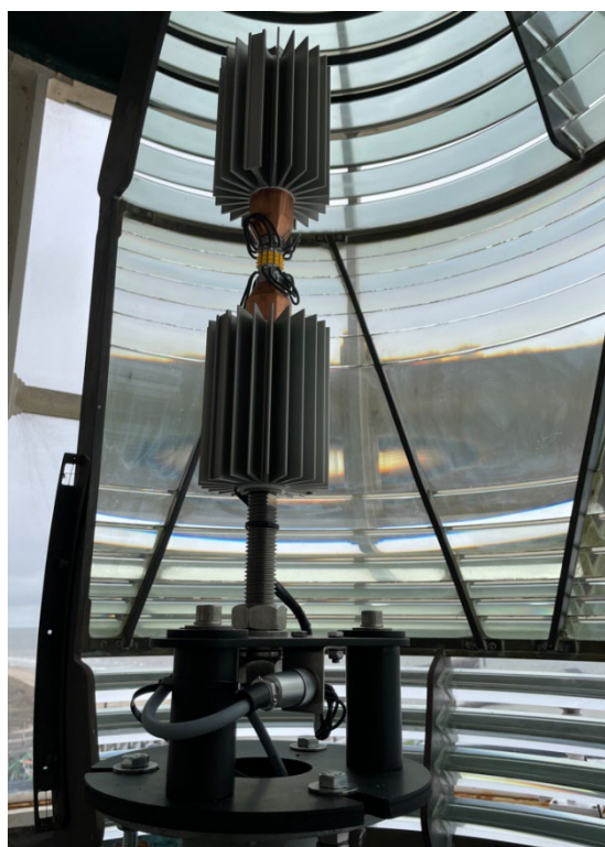
Figure 26: New LED light source Blankenberge
