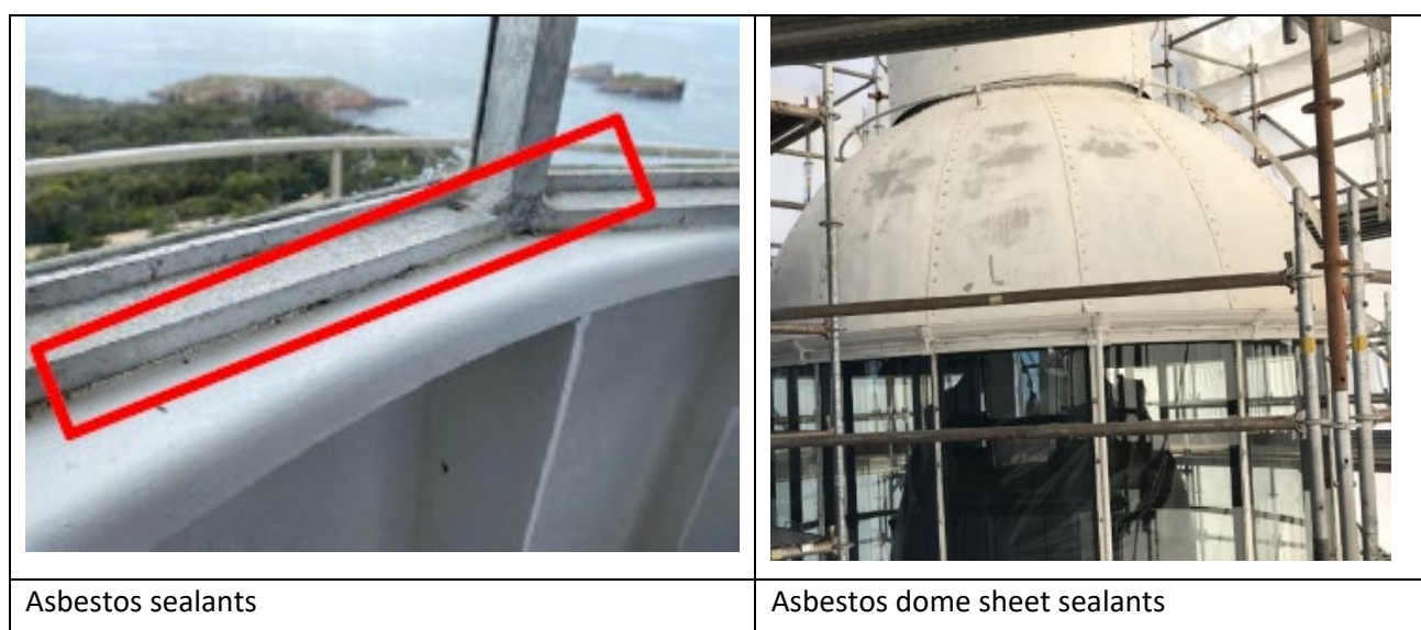
Figure 5: Asbestos examples
