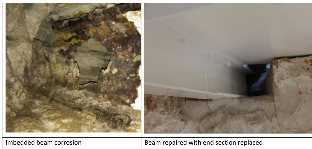
Figure 7: Floor beam repairs
